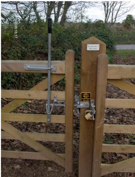
The gate shown opens in either direction and is self closing, fitted with special gravity hinges.
